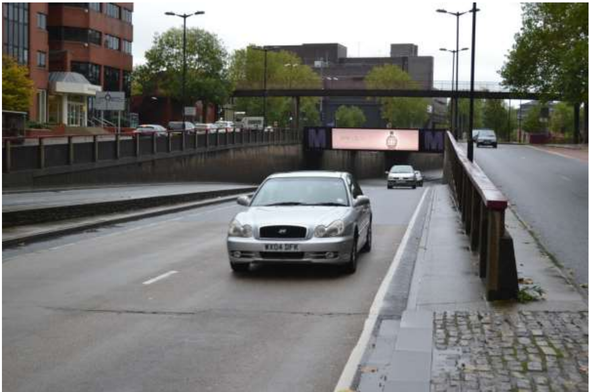
Old Market Roundabout Underpass - Southbound
